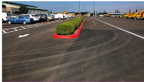
Repaving Project at Saticoy
