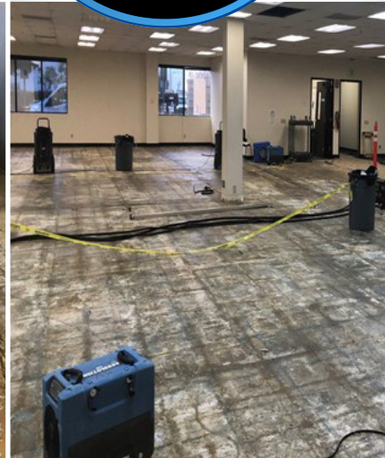
Vanguard Building Remediation
