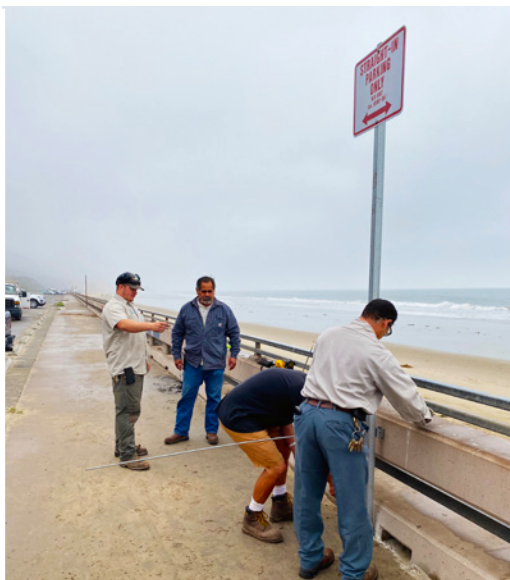
Staff Installing Straight-In Parking Signs
