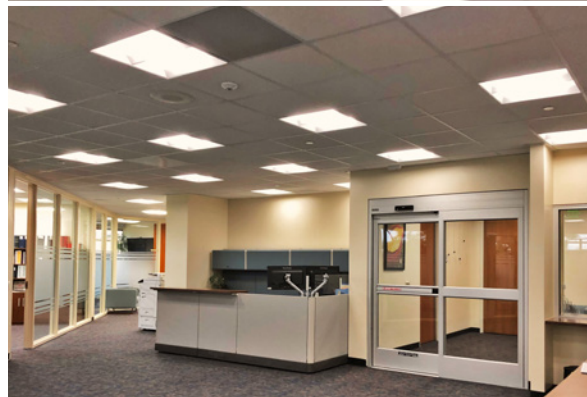
HOA 4th Floor Ceiling & Lighting Replacement
