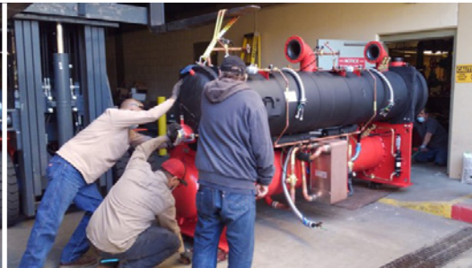
TRJ New Boiler Installation
