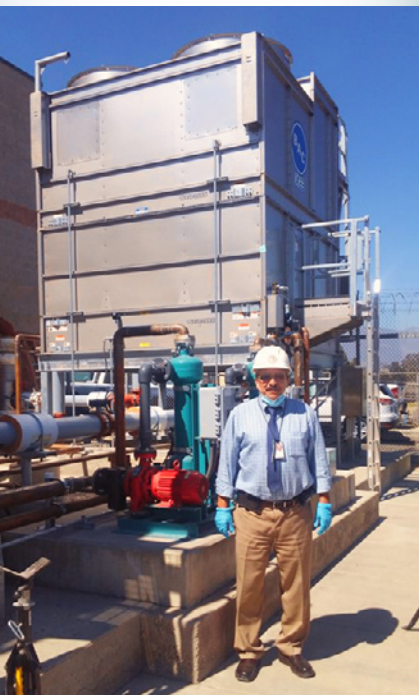
Project Manager Sam Jamshidi at the Cooling Tower Replacement Job Site
